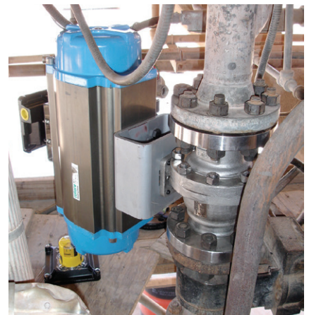
Installed between the lockhopper and lift engager at a major southwest refinery, these 3-inch ASME 300 class metal-seated isolation valves cycle at least three times an hour. These valves replaced another manufacturer's design that lasted only two months.
