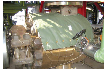
Located in a frigid Scandinavian environment, this large bore ASME 4500 class ball valve is installed on the outlets of the hydrogen heater.
