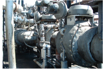
This midwestern refinery has four 20-inch ASME 300 class MOGAS ball valves in overhead vapor service. Several are in their second decade of service.
